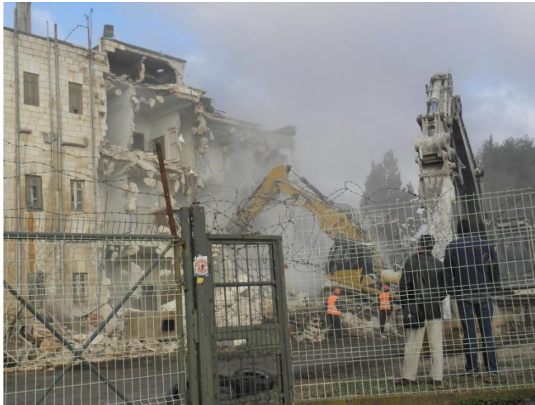
Demolition of Shepherd's Hotel
